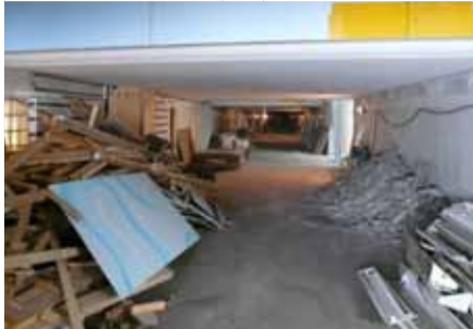
De sloop is begonnen...
